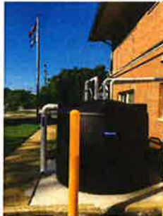
Cistern, Fire Station 206
